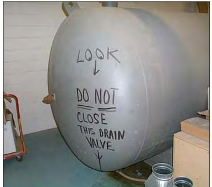
Figure 1: Manual valves left open waste huge amounts of energy.
